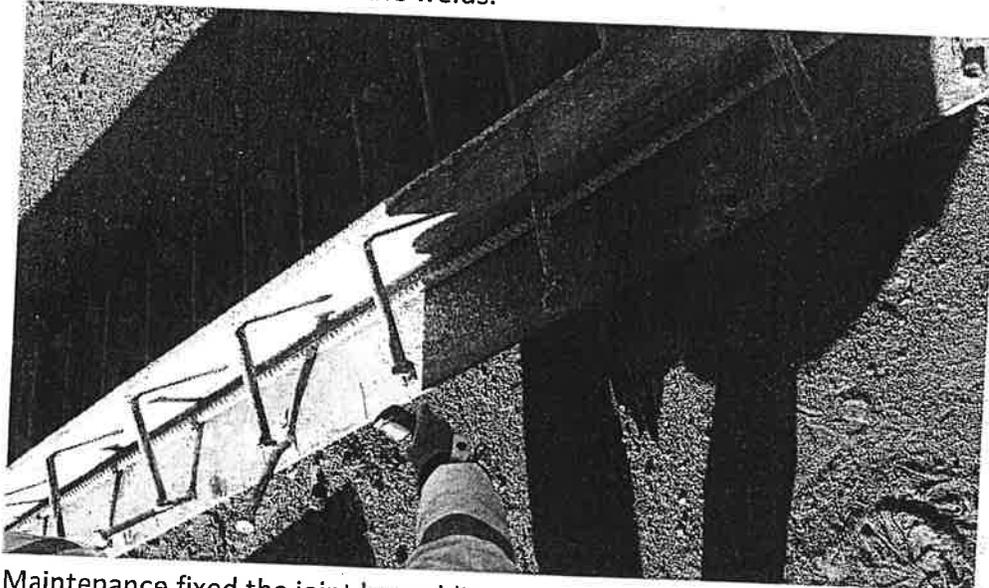
Maintenance fixed the joint by welding more studs on it. There were several proposed long term fixes ranging from require fabricators to use stud guns to changing the Standard Detail to match New Hampshire's or add more studs. The recommended
