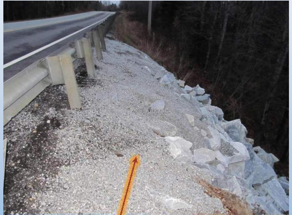
Slope Failure
