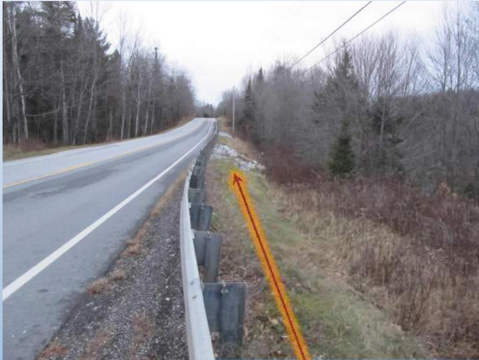
Slope Failure
